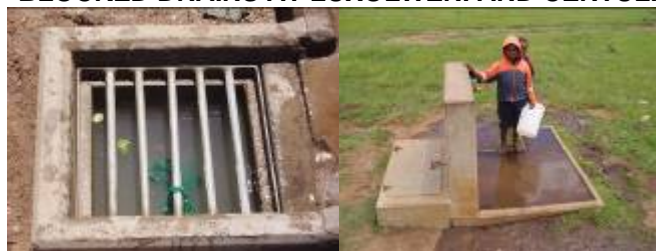
PICTURE 43-44 BLOCKED DRAINS AT LUXOLWENI AND CENTULI
