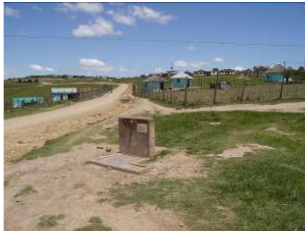
PICTURE 7 ACCESSIBILITY OF COMMUNAL STANDPIPES
