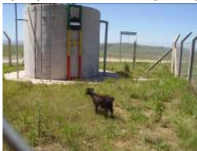
PICTURE 61 FENCING AT WATER RESERVOIRS
