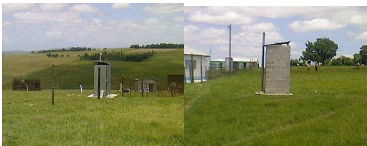
PICTURE 33-34 UPGRADED SANITATION FACILITIES
