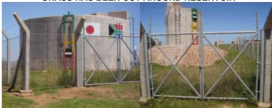
PICTURES 68-69 GRASS HAS BEEN CUT AROUND RESERVOIR
