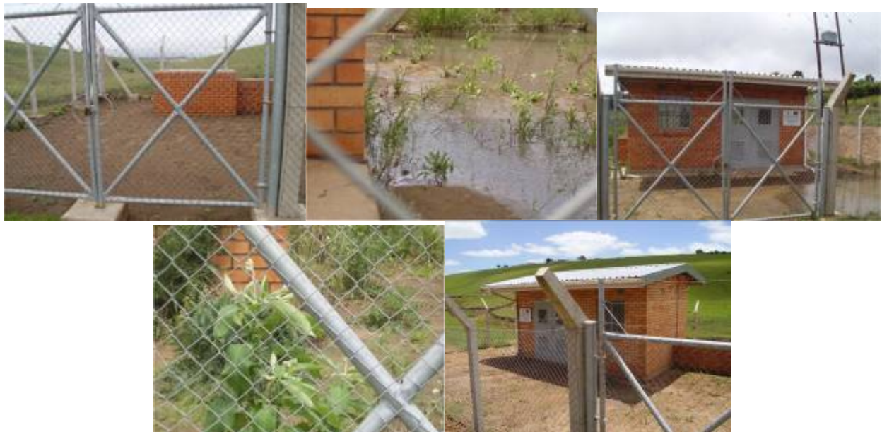
PICTURES 51-55 MAINTENANCE INSIDE
