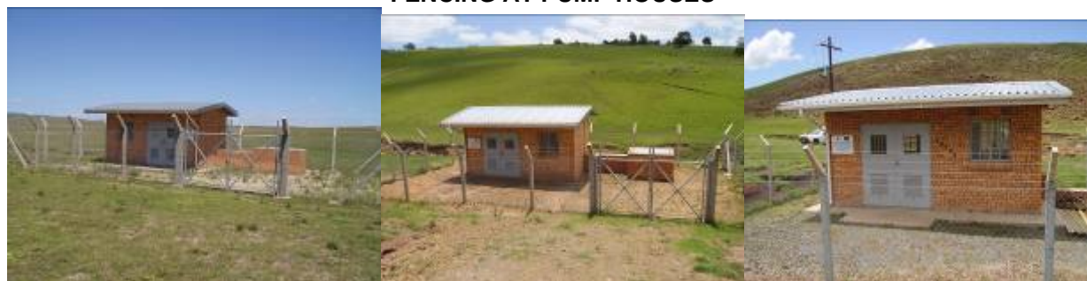
PICTURE 45-47 FENCING AT PUMP HOUSES
